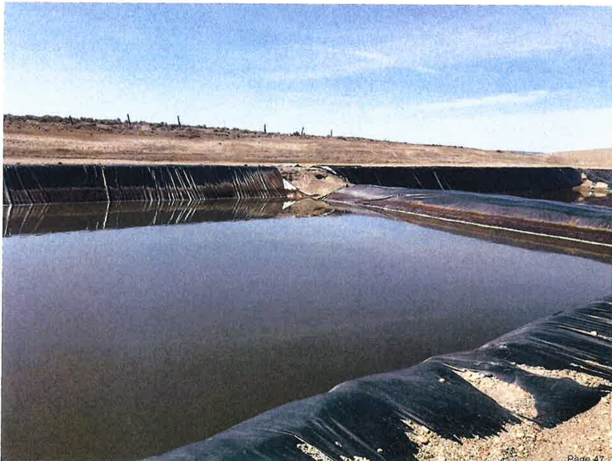
north edge of reserve pit, looking southwest at liner tear
