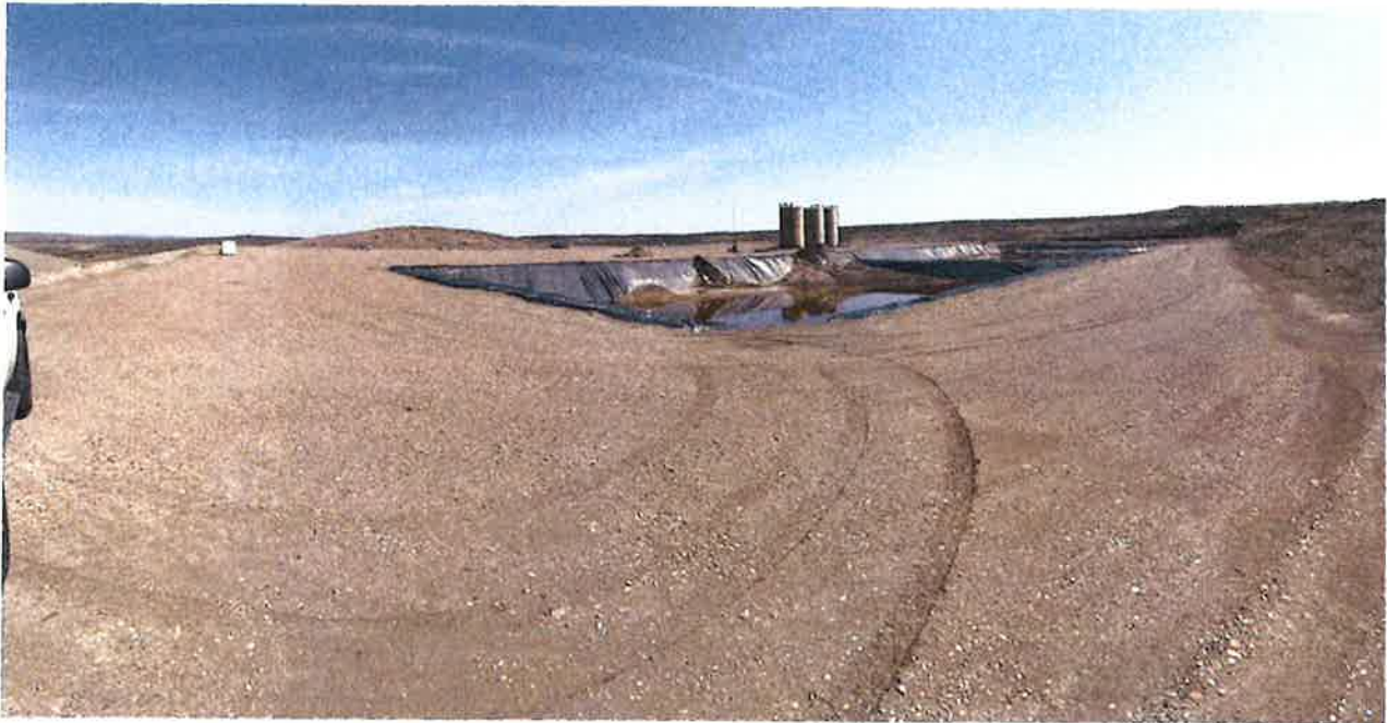
southwest corner of cuttings pit, panoramic looking northeast
