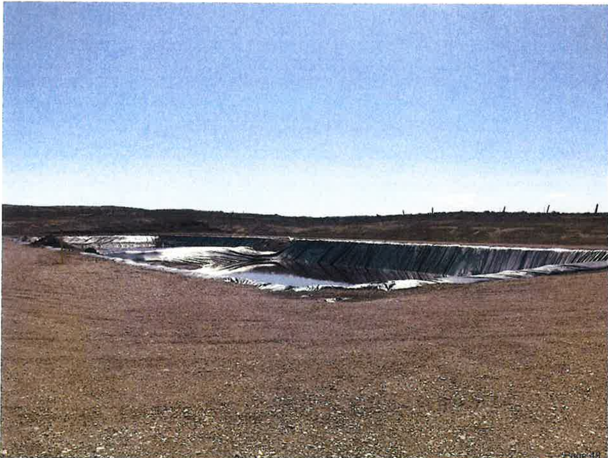
northwest corner of cuttings pit, looking southeast
